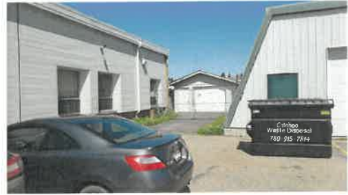
The large footprint that has developed over time has created a large number of alcoves which causes issues for supervision and security.
