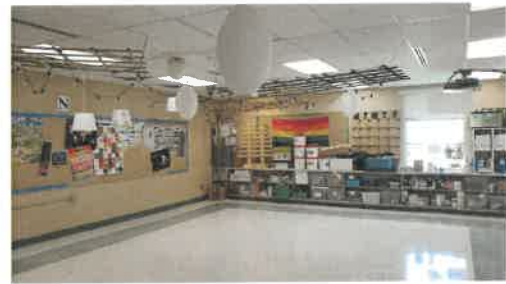
A large number of classrooms have fabric over the light fixtures or have hanging plug-in lamps with extension cords in the ceiling spaces. This is done to provide a variety of lighting levels but is against code and are to be removed.
