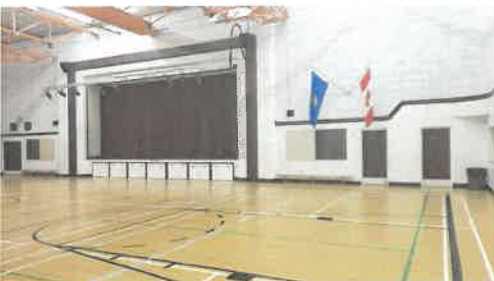
The stage area does not have permanent accessibility and a lift is required to be booked for student access.
