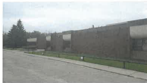
The front lane is able to accommodate the number of buses, but congestion is an issue between buses and vehicles due to the narrow lane width.
