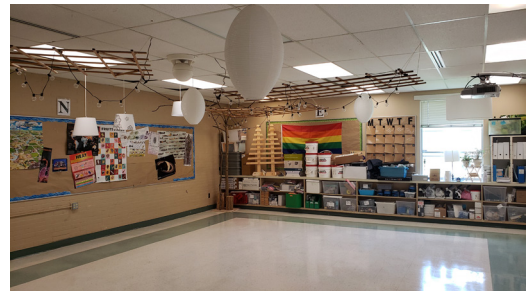
A large number of classrooms have fabric over the light fixtures or have hanging plug-in lamps with extension cords in the ceiling spaces. This is done to provide a variety of lighting levels but is against code and are to be removed.
