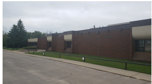
The front lane is able to accommodate the number of buses, but congestion is an issue between buses and vehicles due to the narrow lane width.
