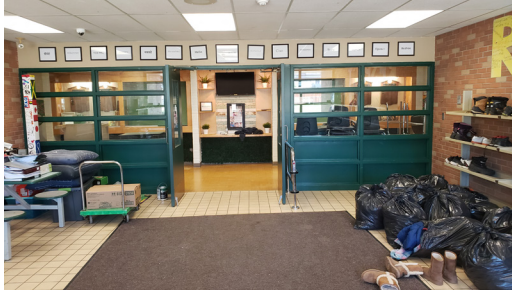
The location of the administration area in relation to the front entrance is good but visibility could be improved to make the entrance more welcoming and improve supervision.
