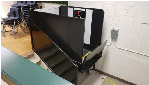
The gym is sunken in relation to the rest of the floor plate. A lift is required for barrier-free access.
