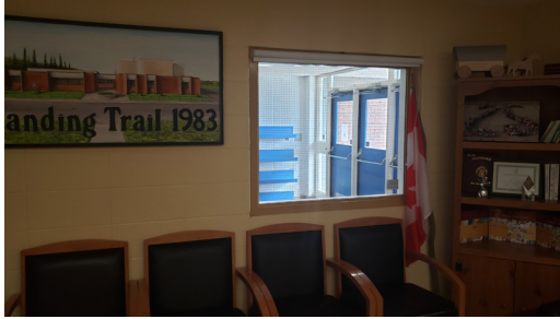
The location of the administration area in relation to the front entrance is good but visibility could be improved to make the entrance more welcoming and improve supervision.
