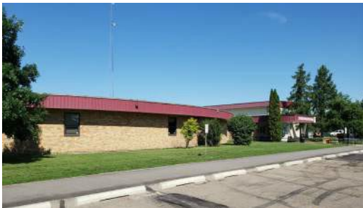
The configuration of the site leads to severe traffic congestion. Accidents have occurred and unsafe parking practices are used. The bus lane is separate from the student drop off area but both lanes use the same exit. In addition, the direction of flow of traffic in front of the school necessitates that students must walk between the cars and across the traffic lane.
