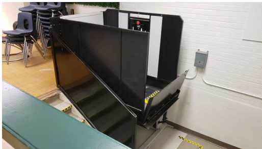
The gym is sunken in relation to the rest of the floor plate. A lift is required for barrier-free access.
