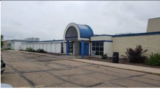
There is confusion about which is the main entrance. Visual cues could be improved such as differentiating the materials at the entrance, moving the school sign closer and installing flag poles.
